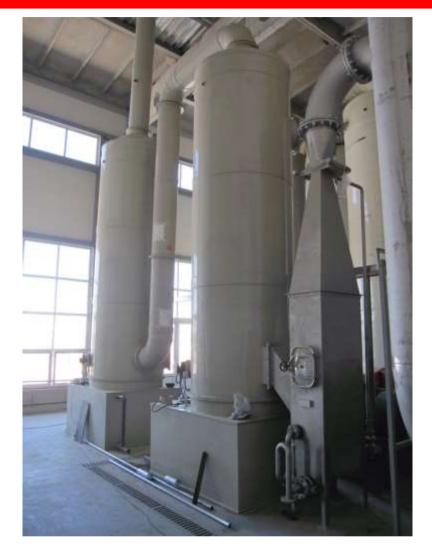
**Function:** Scrubbers, composed of one or more towers, to eliminate volatile organic compounds in the effluents coming from typical rendering processes.
