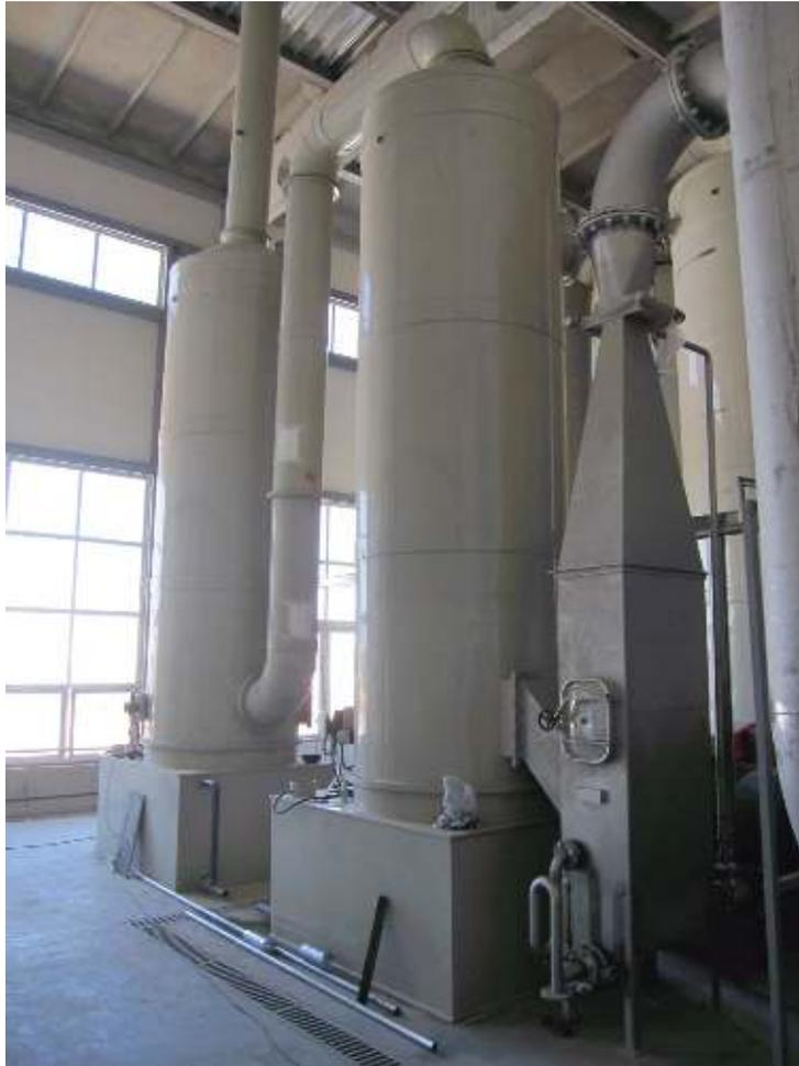
**Function:** Scrubbers, composed of one or more towers, to eliminate volatile organic compounds in the effluents coming from typical rendering processes.
